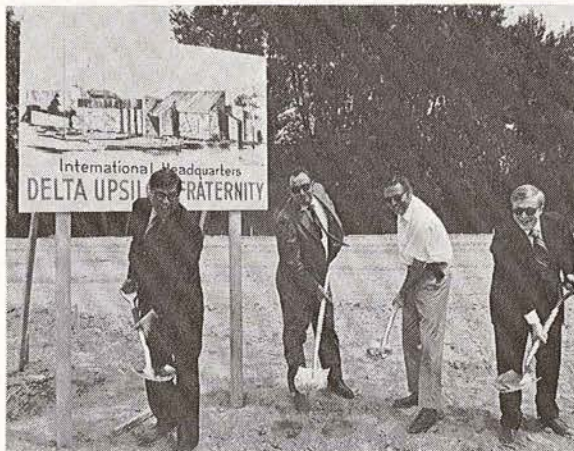
Happy ground-breakers pose before a rendering of the Headquarters building. Left to right, Headquarters Building Chairman Frank B. Jones, Indiana '46 ; Howard R. Peterson, president of Peterson Construction Company; Buert R. SerVaas, Indiana '41 , and Executive Secretary W. A. Butler, Jr.
